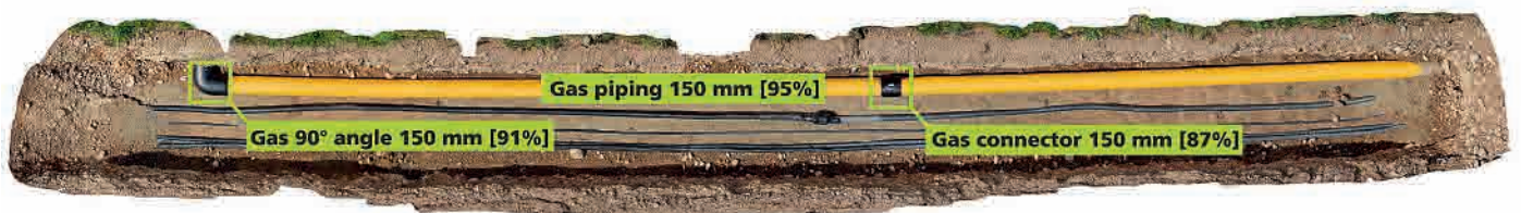
AI-based object recognition software automatically classifies and quantifies infrastructure (diameter of tube in mm, reliability rates in brackets). © Fraunhofer IPM
