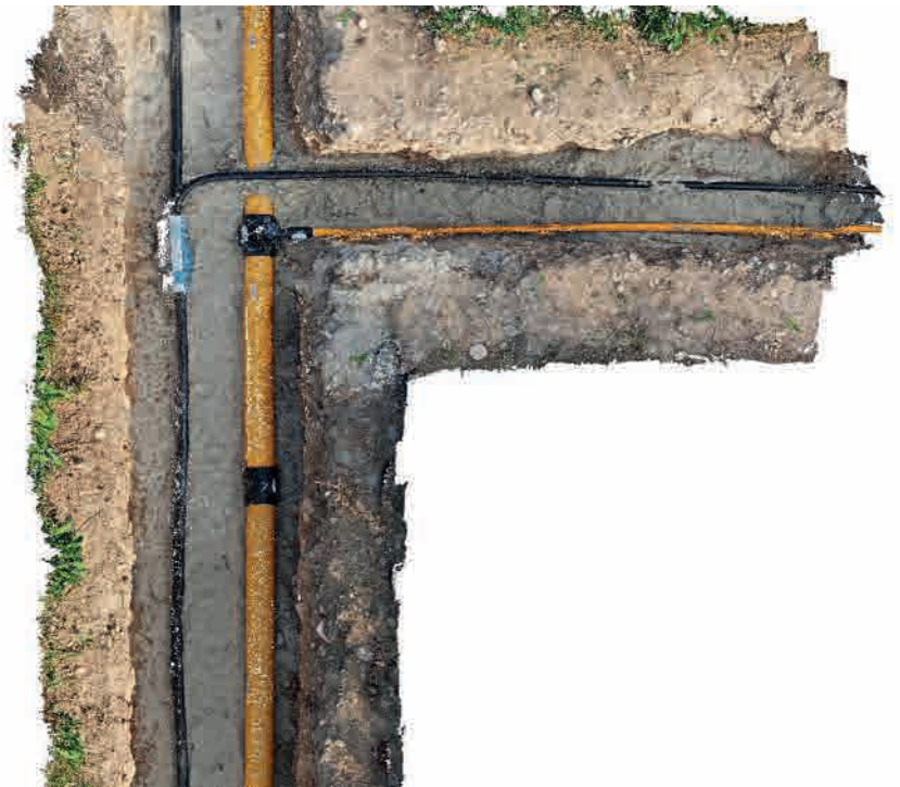
Photo and corresponding point cloud of a building pit. The tube and connectors can be clearly identified in the 3D data. © Fraunhofer IPM
