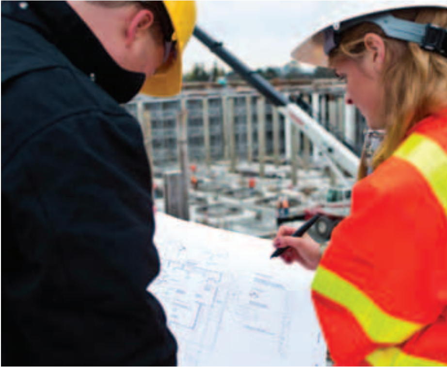
The Digital Pen on site
